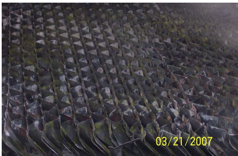
Top-side drift screens on day 41 of the evaluation, cleaned and scale-free due to Micro-Nice® D-5's action through tower sprays with no hosing or power-washing.
