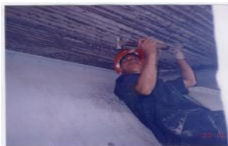
Cracking out Scale
